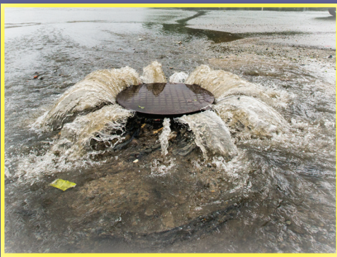
Odors from sewer mains & sewer overflows.
