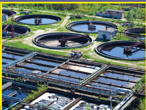
Odors found anywhere at the WWTP.
