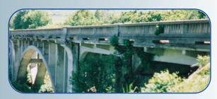
Salt and chlorides used to de-ice roadways fall from bridge decks, rusting and corroding expensive underbridge components, such as rocker arms and concrete support pilings.
