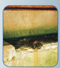
Concrete is slowly eaten away by the salts and chlorides exposing rebars and greatly reducing the structural integrity of the piling component.
